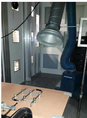
Figure 1. Diffuser pipes with capture hood inside particle free test chamber
